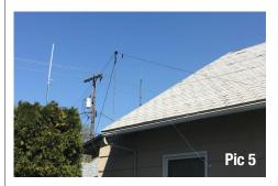
**Pic 5** is another mast shot taken before I secured the 20m wire that I had to raise the end point on as it was at too tight of an angle.
